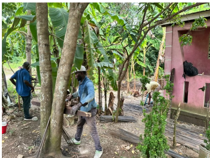
Working with Rebar in Front of Storage House.
