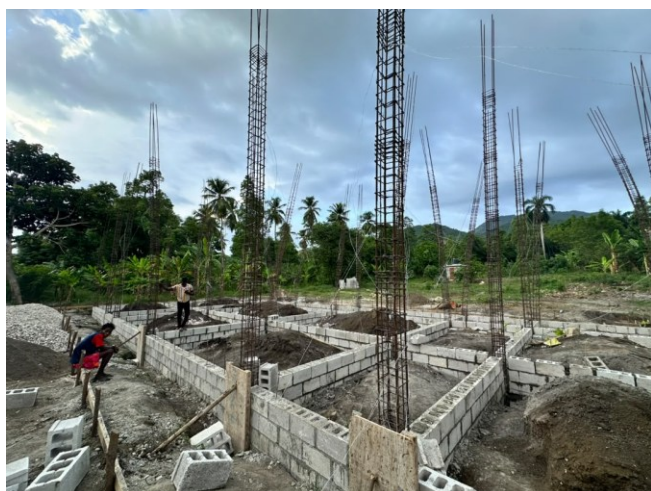
Third Row of Block Completed
