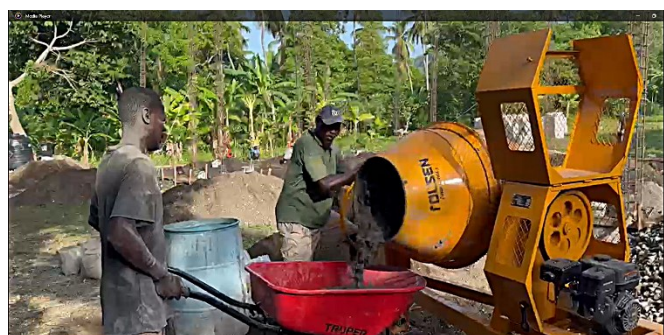
Pouring the Concrete Footer
