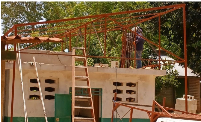
Installing Solar Panels
